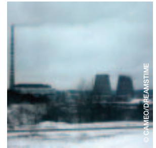
image A power generation plant near Vilnius, Lithuania on a cold winter's day.
