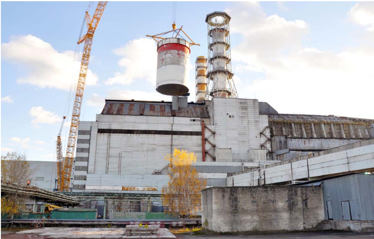
Fig. 35 The shelter "sarcophagus" built on Unit 4. (source chnpp.gov.ua)
