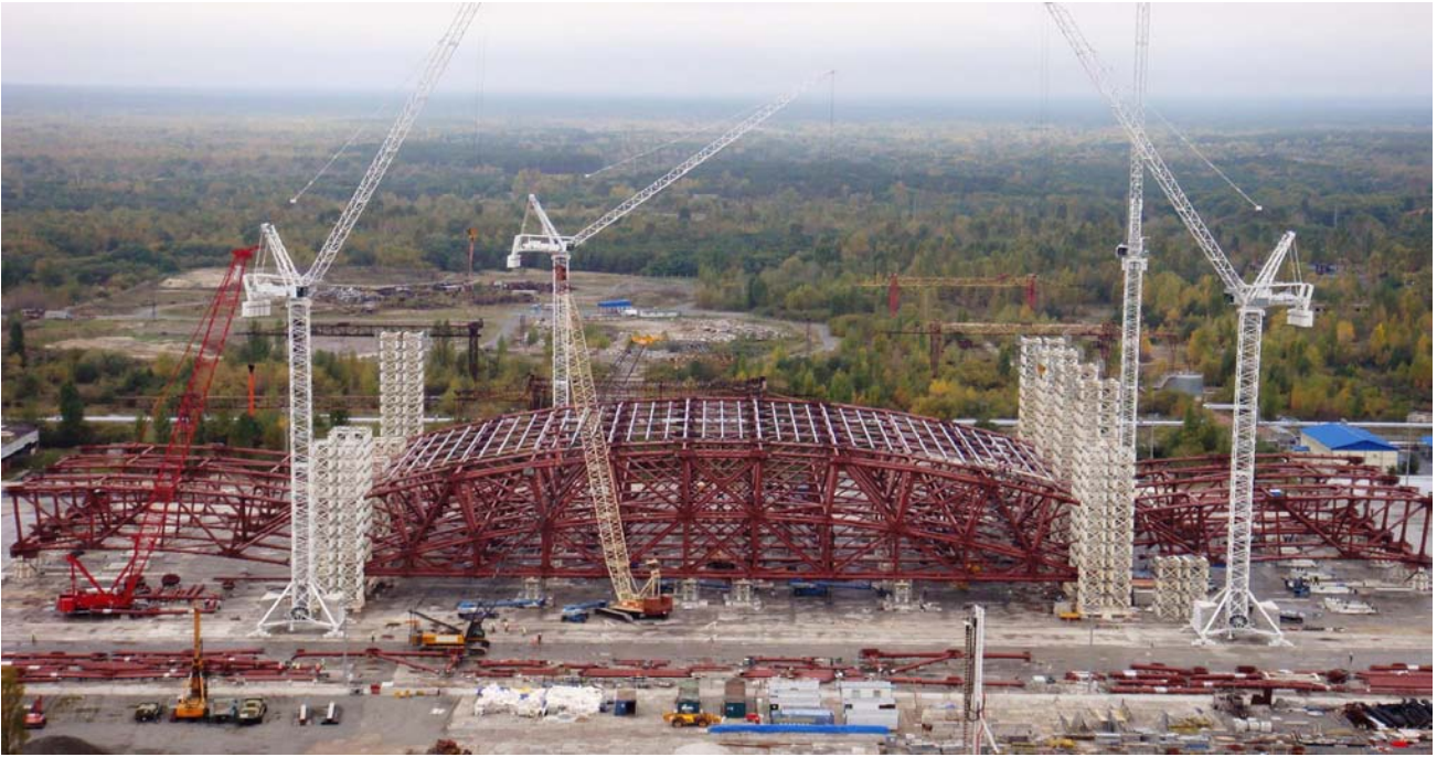
Fig. 38 Initial assembly first bay structure (source chnpp.gov.ua)
