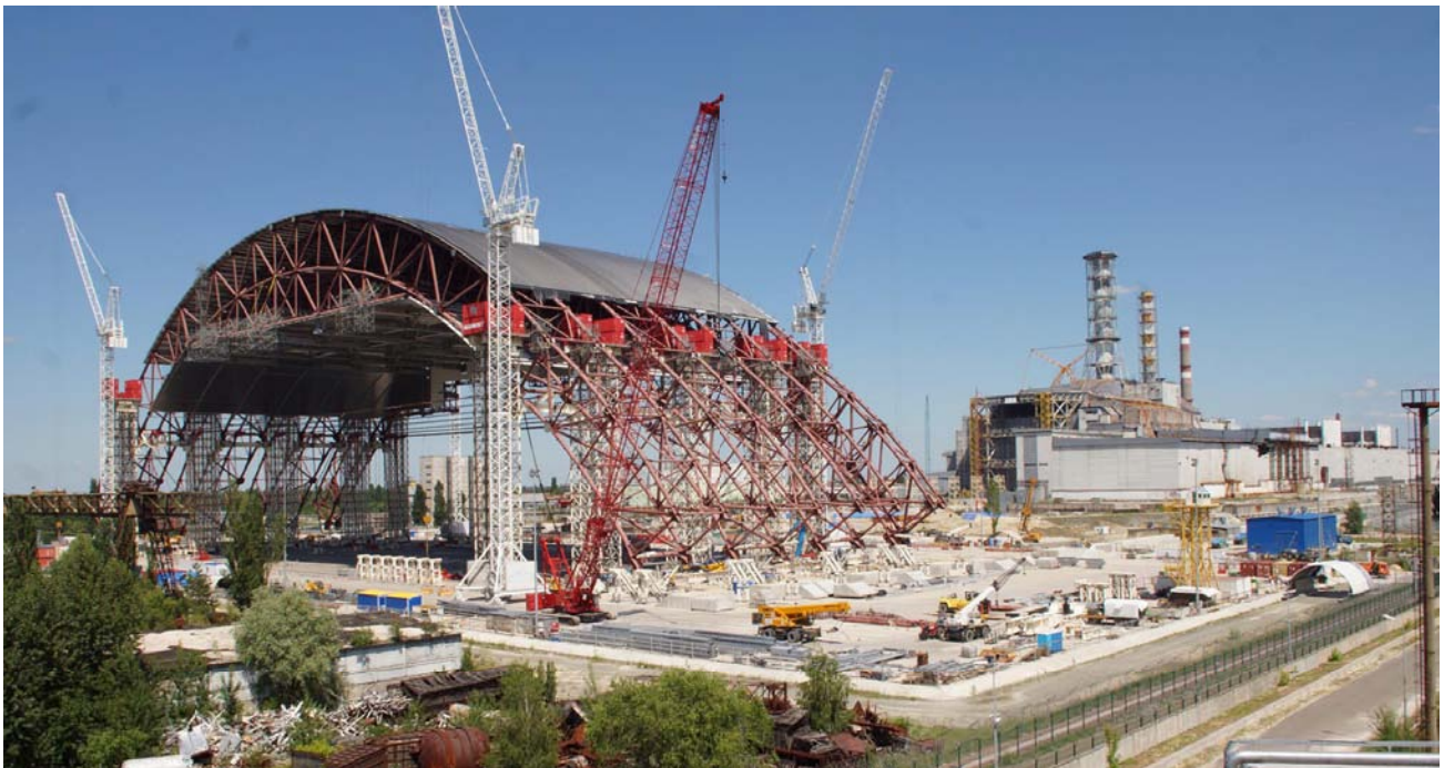
Fig. 40 Assembly first bay structure (source chnpp.gov.ua)
