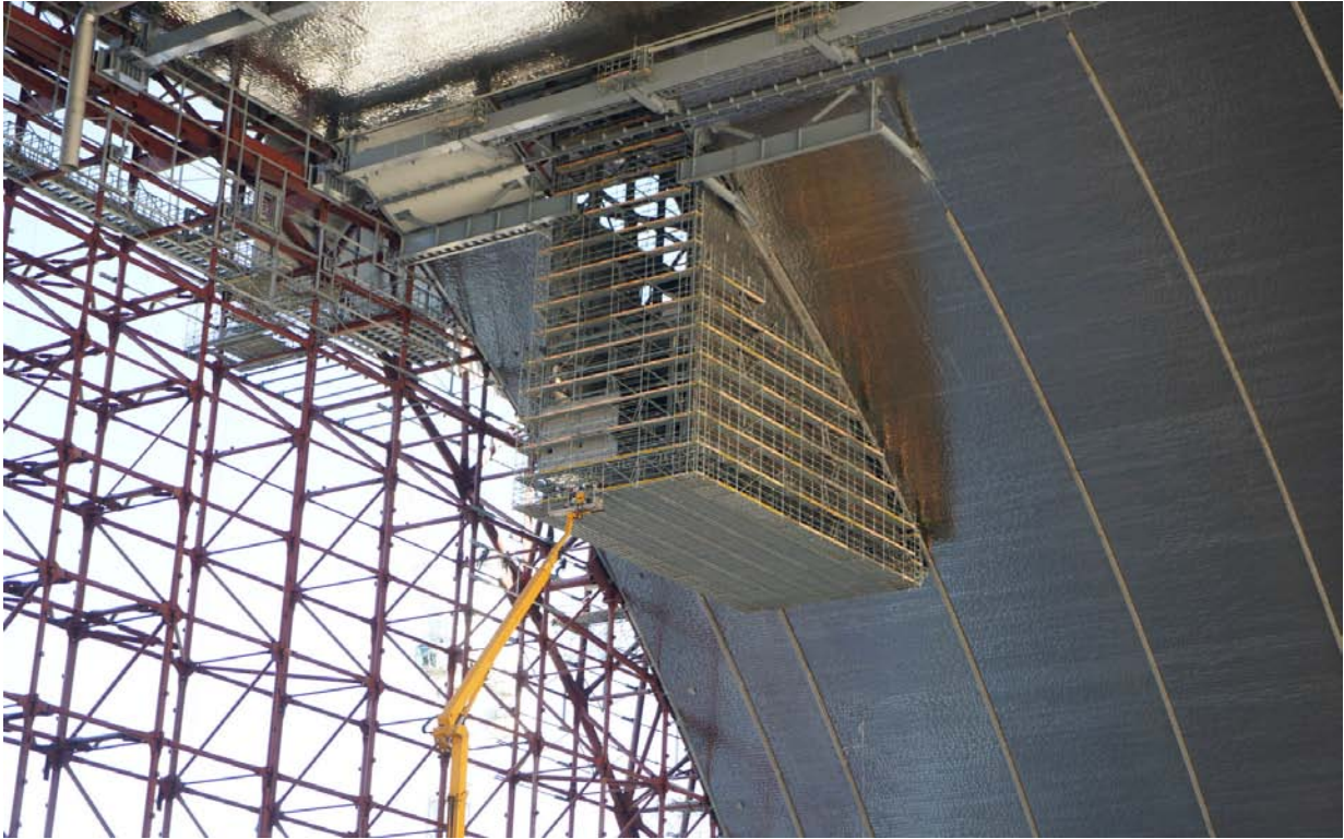
Fig. 47 Assembly of internal surface (source chnpp.gov.ua)
