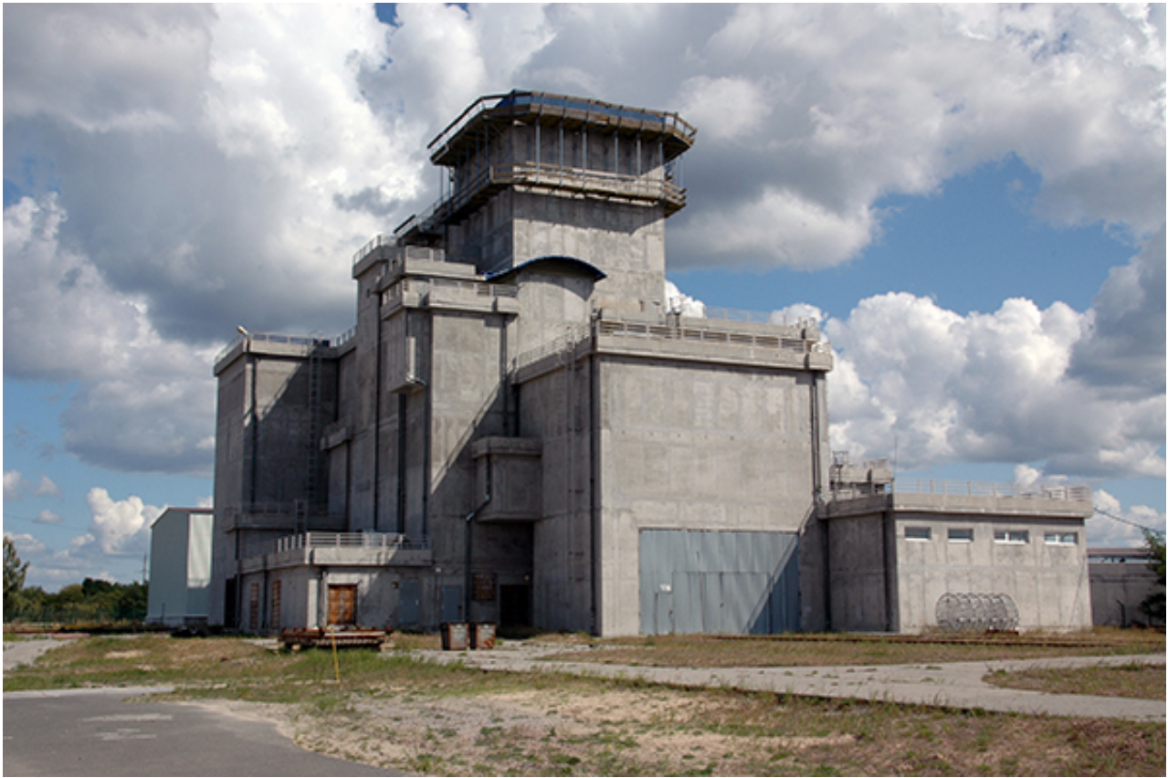
Fig. 23 The ISF-2 Processing Building (source chnpp.gov.ua)
