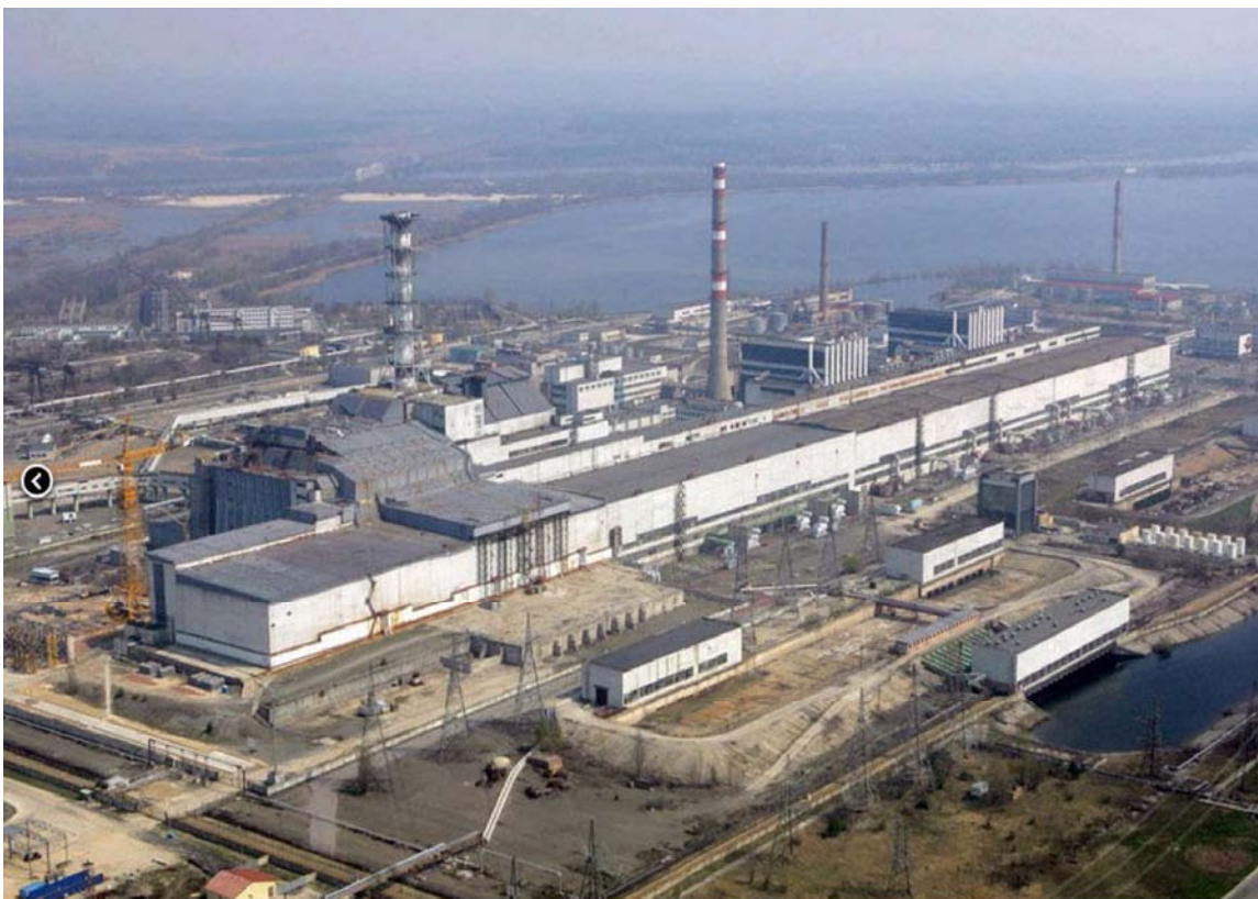
Fig. 16 View of Chernobyl plant following the completion of "sarcophagus" (source: chnpp.gov.ua )
