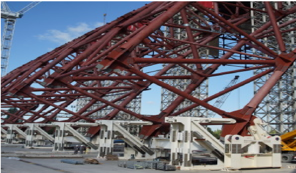
Fig. 42 Details of arch supporting structures bases (source chnpp.gov.ua)
