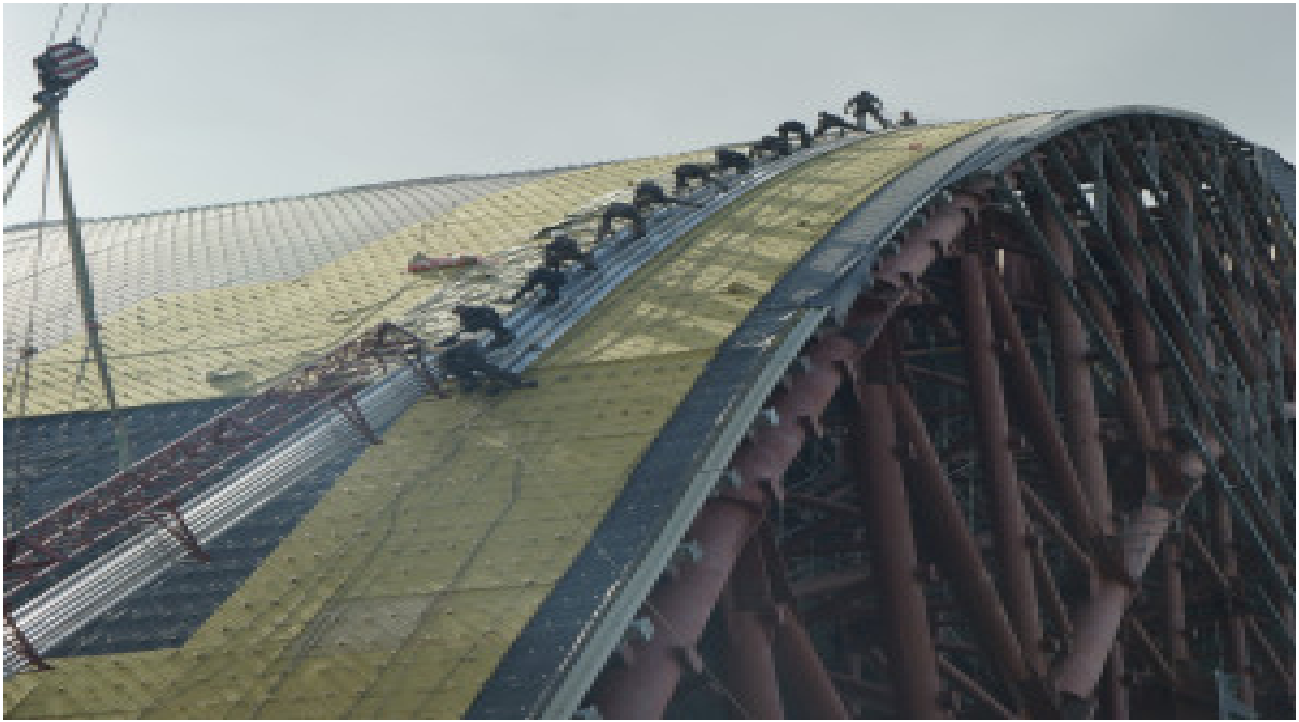
Fig. 46 Details of roof (source chnpp.gov.ua)
