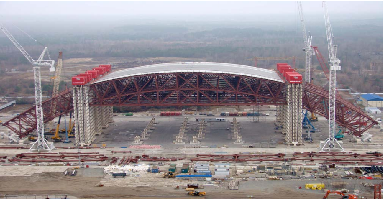
Fig. 39 Initial assembly first bay structure (source chnpp.gov.ua)
