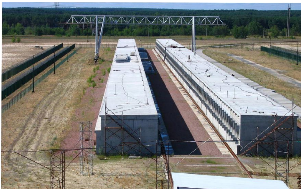
Fig. 30 The Fuel Storage area consists of 58 concrete storage modules (CSM) with 4 cells each - 232 cells in total, (source Holtec)
