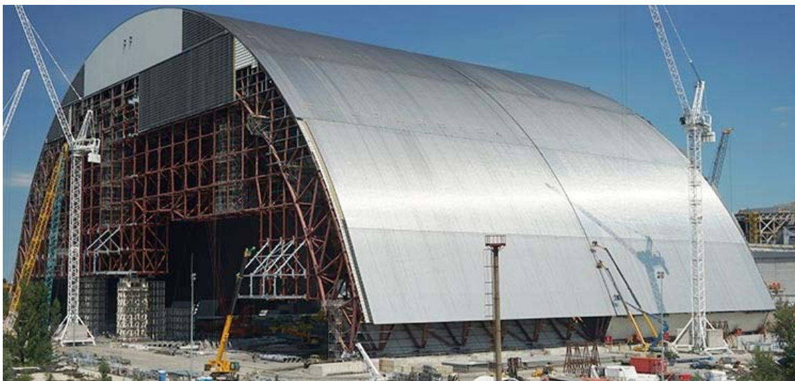
Fig. 49 Assembly the of two sections (July 2015) (source chnpp.gov.ua)
