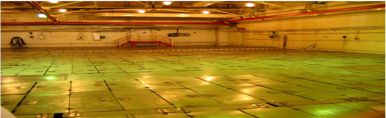
Fig.17 The Interim Spent Fuel Storage ISF-1 (source: chnpp.gov.ua)
