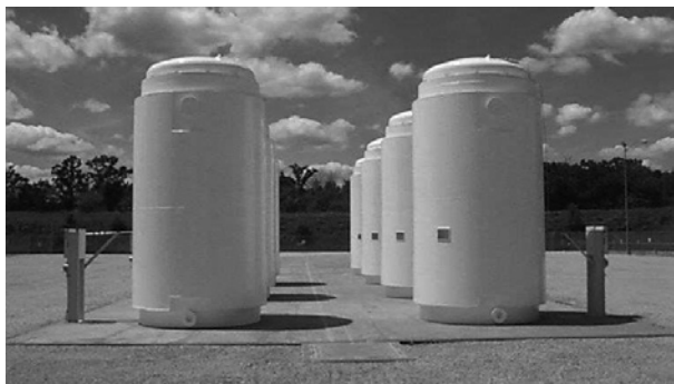
Dry casks used to store spent fuel
